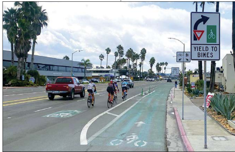
An example of a Class 2B bike lane on Coast Highway, Encinitas.
