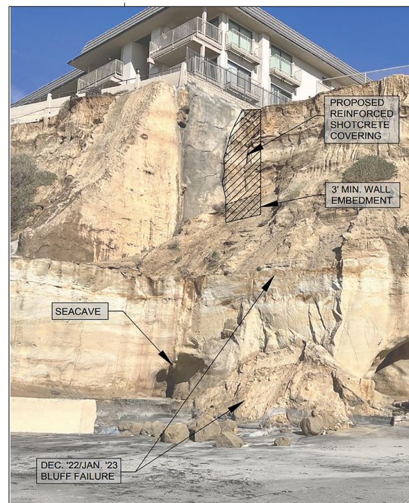
Details of repairs
