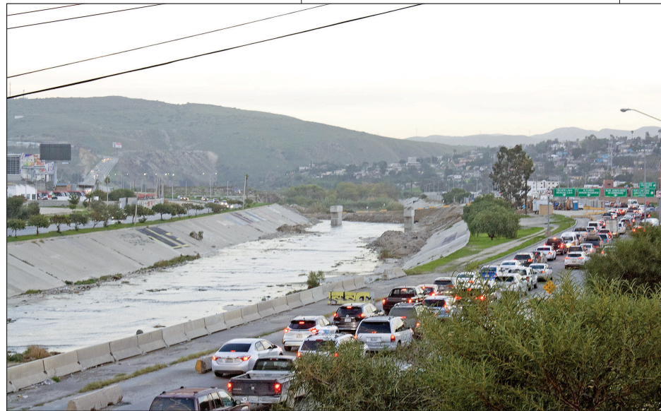
Without the bridge and the embankment, the usual 25-minute trip has turned into 90 minutes or more.
