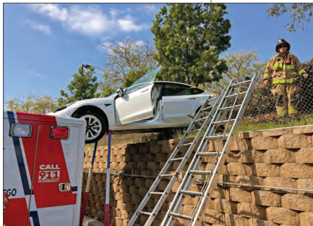
The fire department noted the "stacked stone wall" was "not a masonry wall, so the integrity is at risk."
