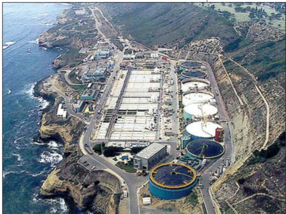
Point Loma wastewater plant.
