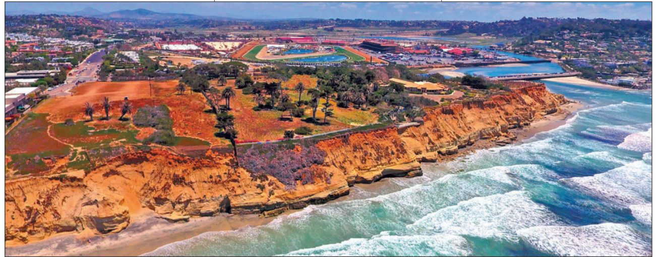
A 16-acre plot of land West of the Fairgrounds showing coastal erosion and collapse.
