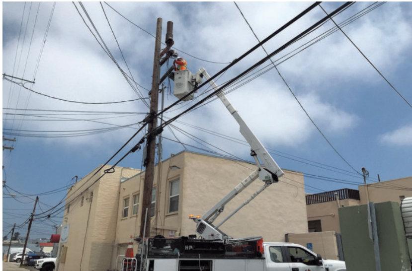
Jeff attaches cables. Above him, the 4G transmitter cell he is installing. Is the apartment below safe?
