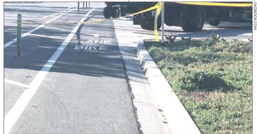
Forcing a truck to cross and block a traffic lane as it makes a right turn seems...inadvisable.
