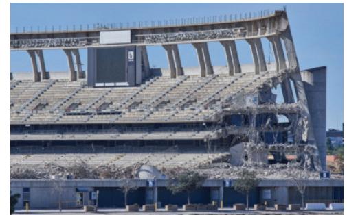
Capturing a week's worth of progress in the demolition.
