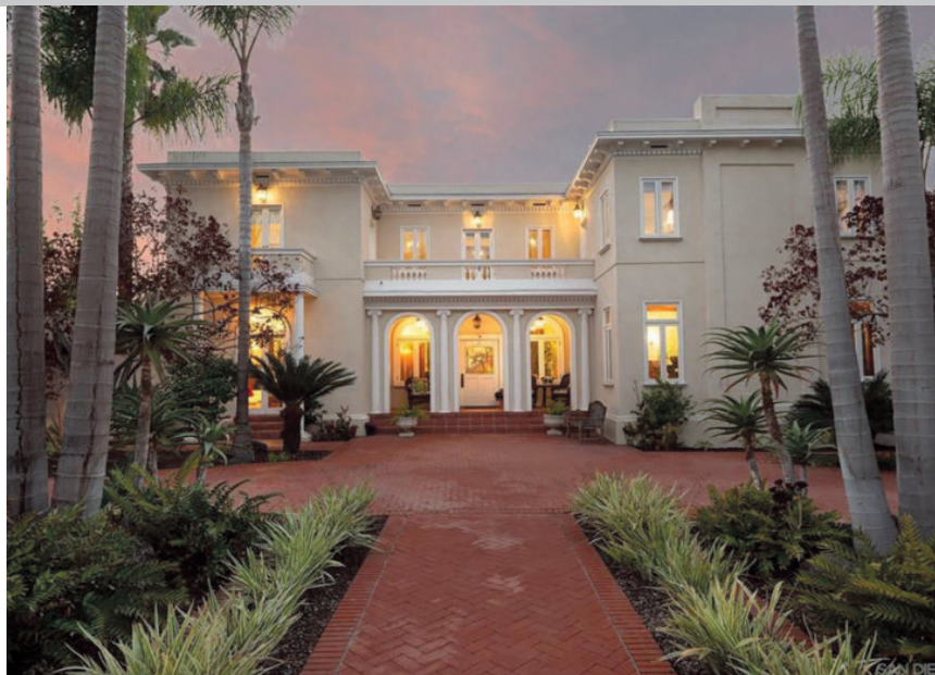
Square Ionic columns! Cornice molding! Bracketed dentils! No wonder the architectural sketches made the local paper! (Also, the owner was the editor.)
