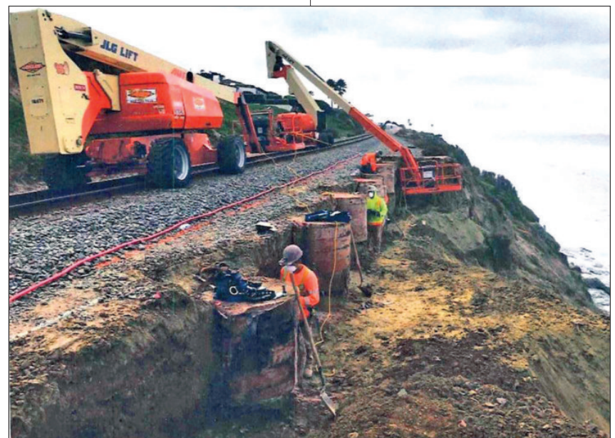
Repairs in process.
