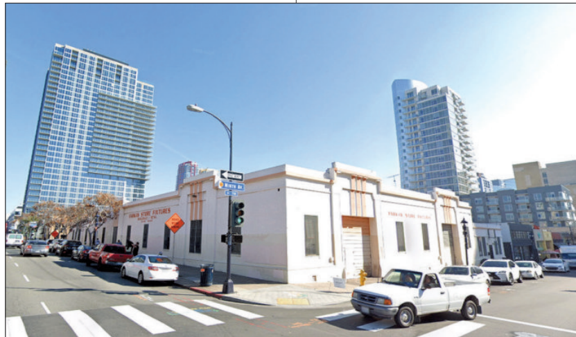
The new above-ground parking levels will rest atop the old structure.
