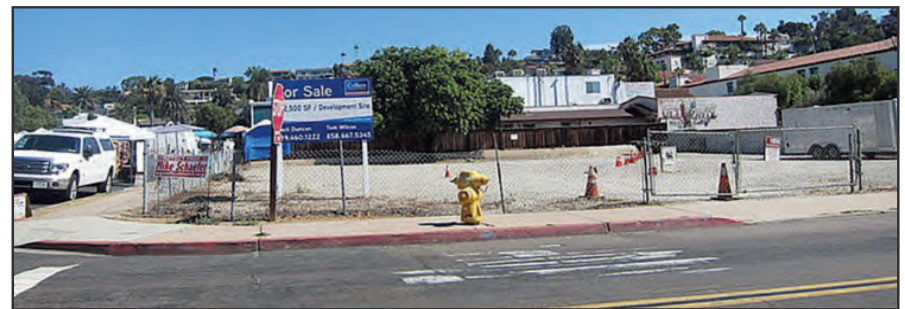
This vacant lot at Congress and Harney Streets in Old Town will become a 43-space paid parking lot before eventually becoming the site of new apartments.
