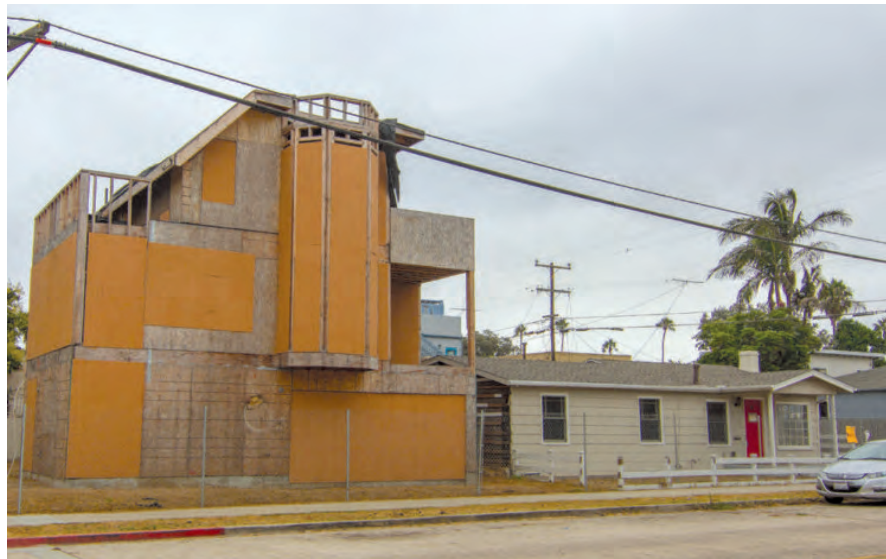
The original four-bedroom, two-bath home (right) and the expansion.
