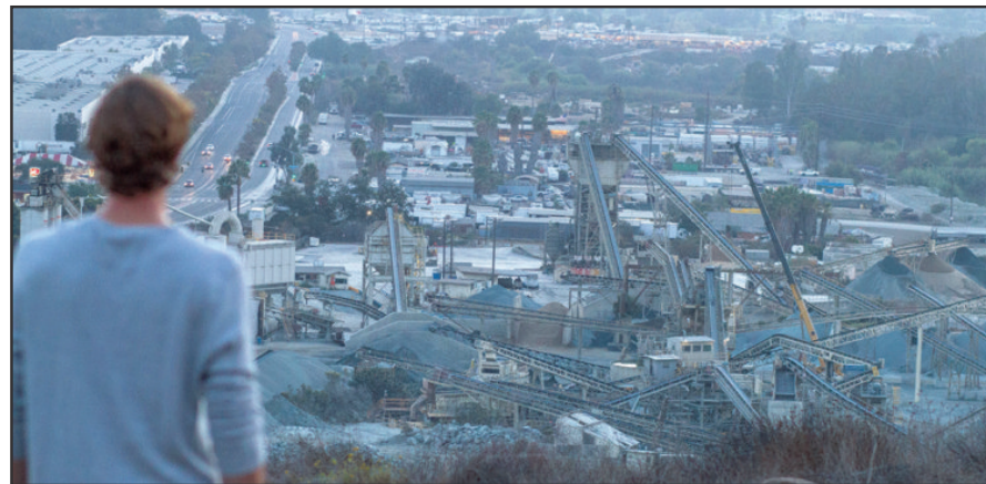
A neighbor looks down on the Superior Ready Mix operation from a hillside to the east. Mission Gorge Road is on the left.
