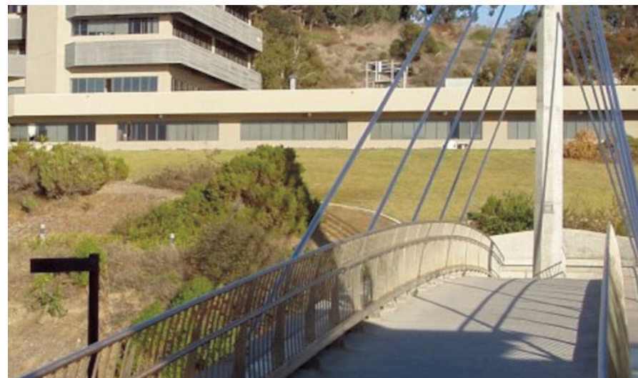
Pedestrian bridge — you have to climb several dozen stairs (or take a very slow elevator).
