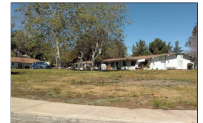
Peñasquitos Village: conditions indicative of a property soon to face the wrecking ball
