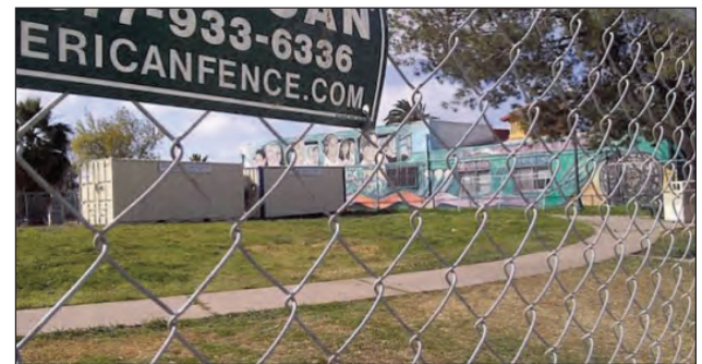
Adams Avenue Elementary construction yard: “This really shows a lack of respect to the many area residents that use the park.”
