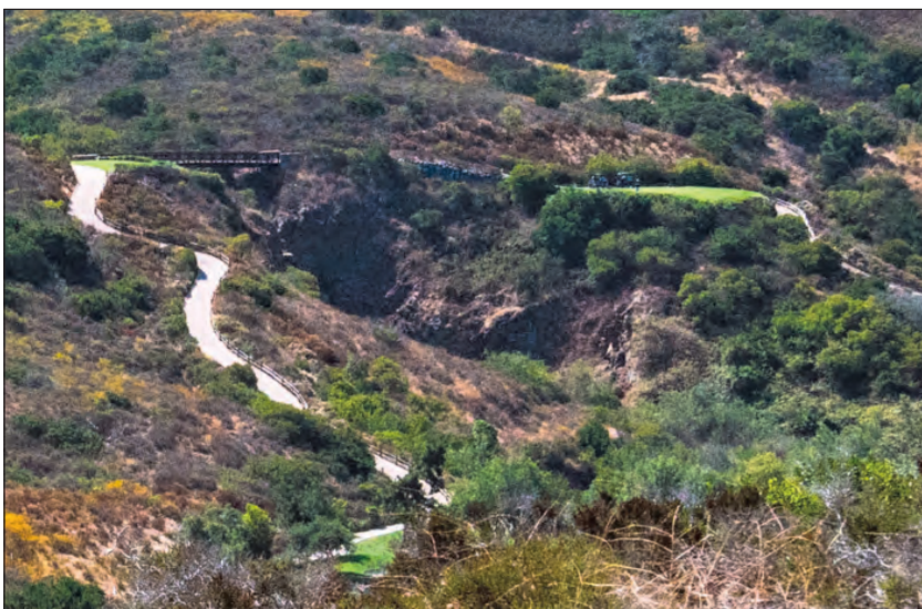
The bridge crossing Macario Creek (upper left)
