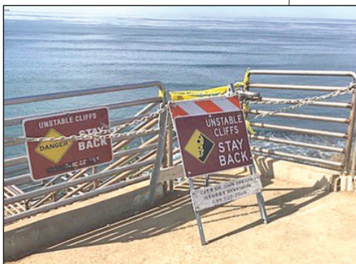
Ladera Street stairway. Access to North and South Garbage difficult...go surf O.B.
