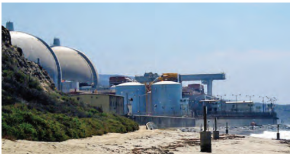
Edison made fast transfer of nuclear waste into dry casks.
