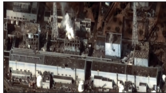
The Fukushima Daiichi Nuclear Power Plant after the 2011 Tohoku earthquake and tsunami
