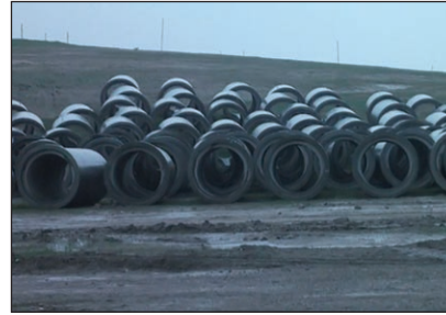
Sections of culvert to be used in border-crossing construction
