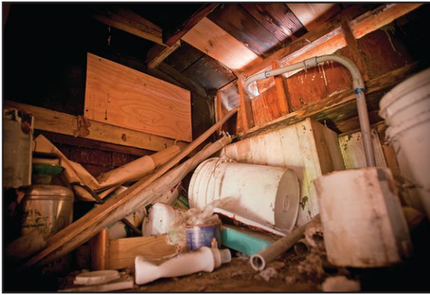
Plywood covers the area where raccoons entered the attic.
