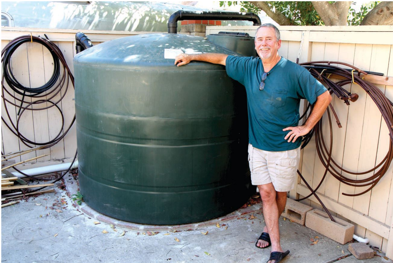
Bob Greenamyre's 1000-gallon water tank fills up from his roof gutters after a total of four inches of rain has fallen.
