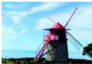
BonnieMaffei: Windmill, used to grind corn, constructed with lava rock, Island of Pico, Azores
