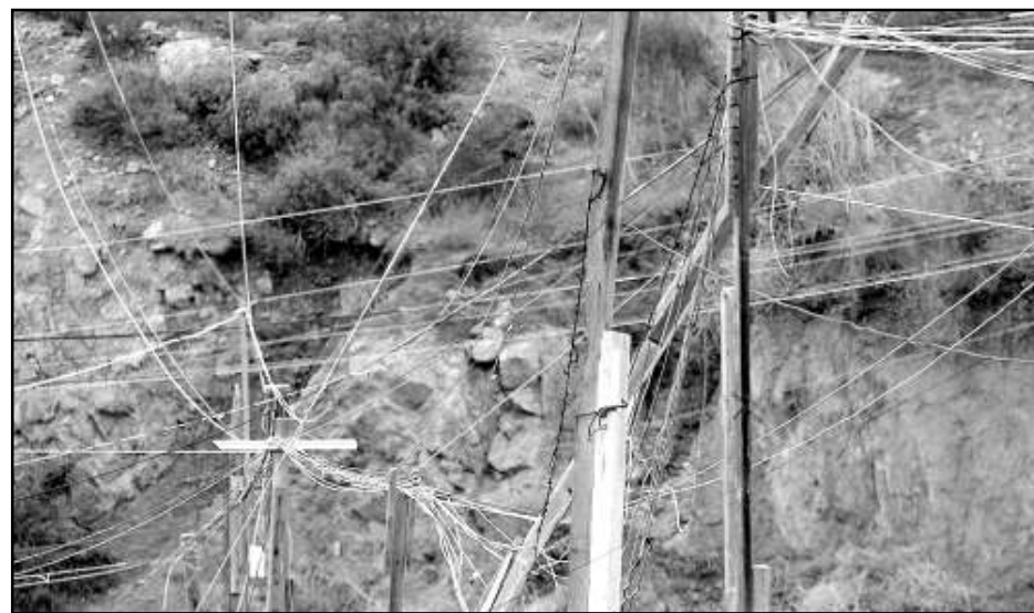
Illegal power connections, eastern area of Tijuana
