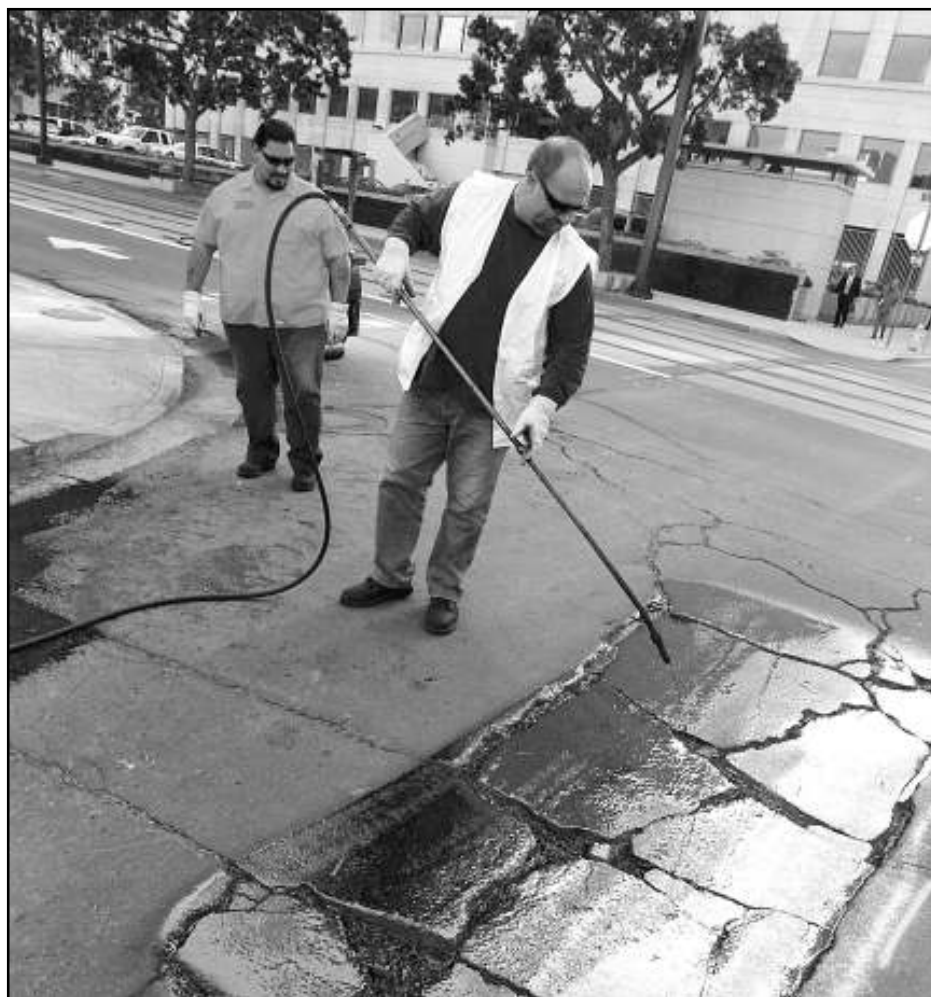
Pothole sprayed with emulsion bonding agent
