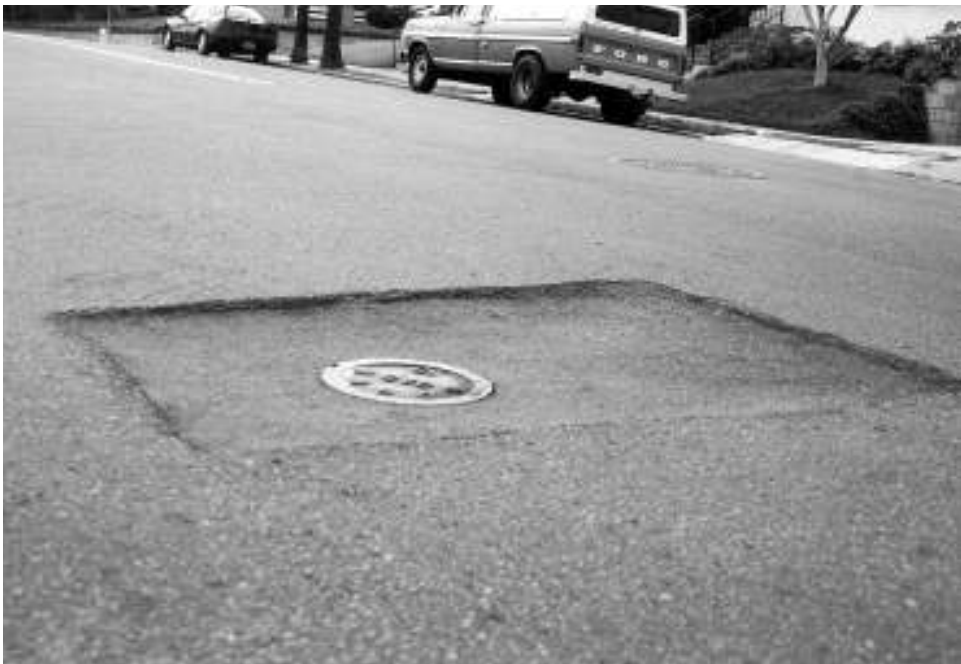
Sunken trench surrounding gate valve cap, Sutter Street
