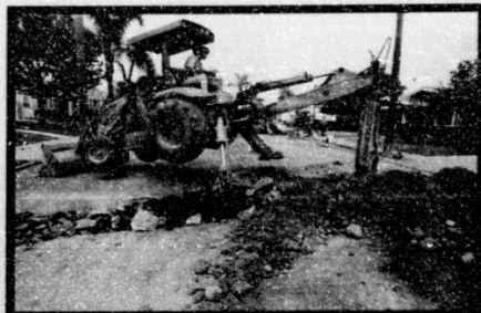
Mark Breckner on a backhoe fitted with sheep's foot
