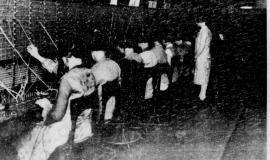
Pacific Telephone switchboard room, and end of a long-distance call; the switchboard iself was called a "multiple" in which and satellite links, communications operators plugged "jack cords" into any one of thirsty San Diegans placed their messages
