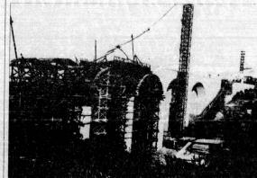
abrillo Bridge under construction, circa Cantilever type bridge was built across 1914 California's first multiple-arched then-Pound Canyon (later renamed Cabrillo Canvon) by Frank P. Allen at a cost of \$214,000. Cabrillo Bridge has been the launching site for The structural engineer for the bridge was numerous "jumpers" leaping to their deaths Thomas B. Hunter, an employee of the California Division of Public Works.
