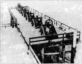
These Rube Goldberg-looking contrap-tions are actually "wave motors" installed on the end of an Imperial Beach pier, circa 1912. They were the brainchild of Charles E. Edwards, a San Diegan who envisioned harnessing the action of the waves that rolled in beneath the pier to generate electricity for the residents of "South San Diego Beach" (as I.B. was then known).
