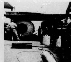
Decompression chambers on construction barge
